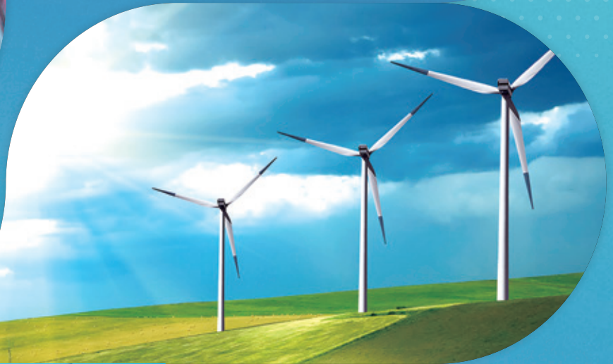
• Wind Power Automation Control Solution
